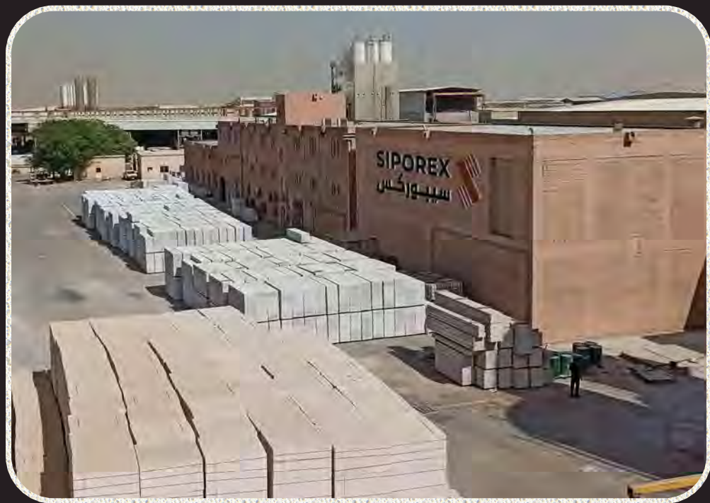
Siporex manufacturing plant in Riyadh, Saudi Arabia
