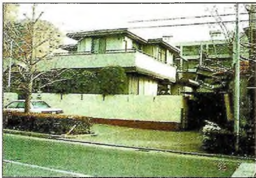
ALC Bldg. aftermath of quake
