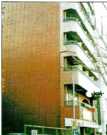
ALC exterior wall of mid-size office building : degree I
