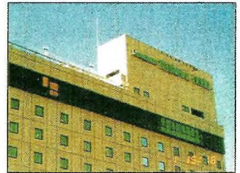
ALC Penthouse atop a terminal building (Degree A)
