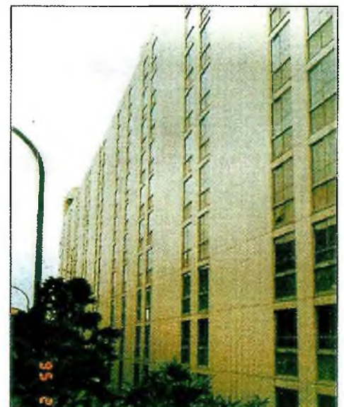
ALC wall of mid-size mansion : degree I
