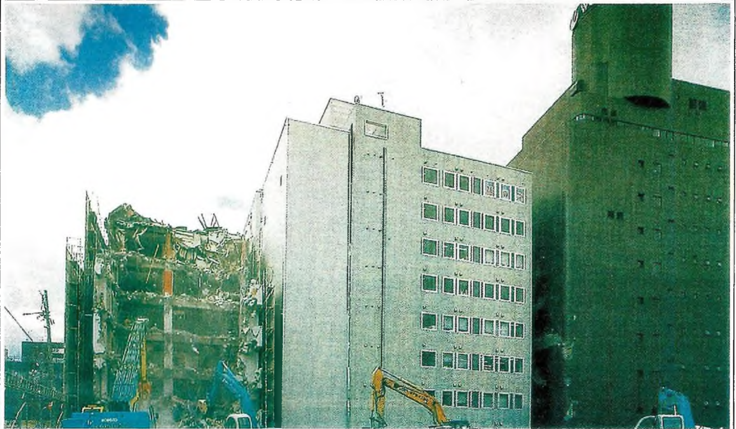
The structure built with ALC Quake - resistance property stands intact with adjacent building seen in total destruction.
