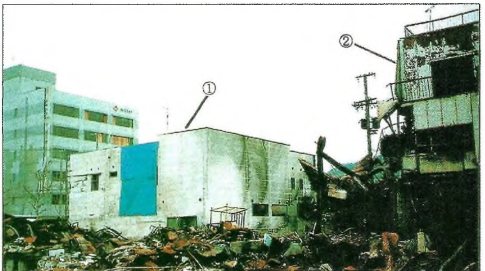
2 ALC Building with gutted interior. ALC Bldg. 1 partially burned is still standing
