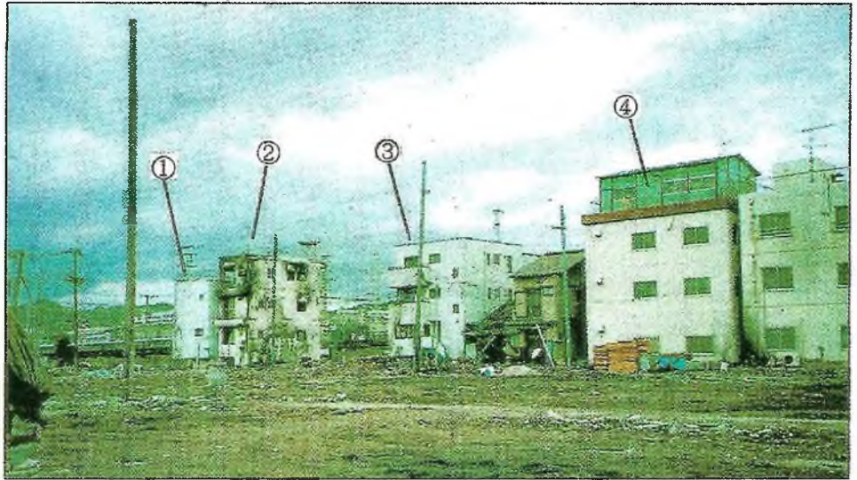
Surrounding area completely gutted. Note that a wooden house between 3 and 4 is burned down ALC Bldg. 1 & 2 are standing intact.
