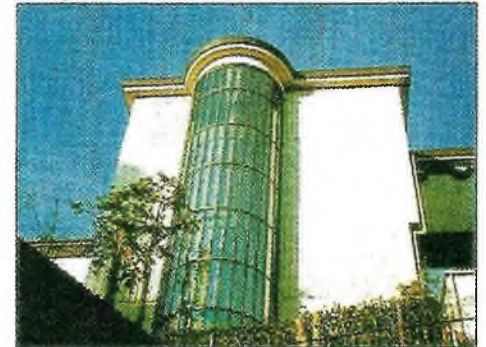
4 storey ALC building, clinic/resident's : degree A
