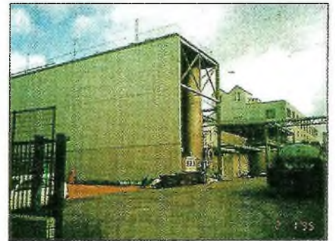
ALC Exterior wall of a plant (Degree A)
